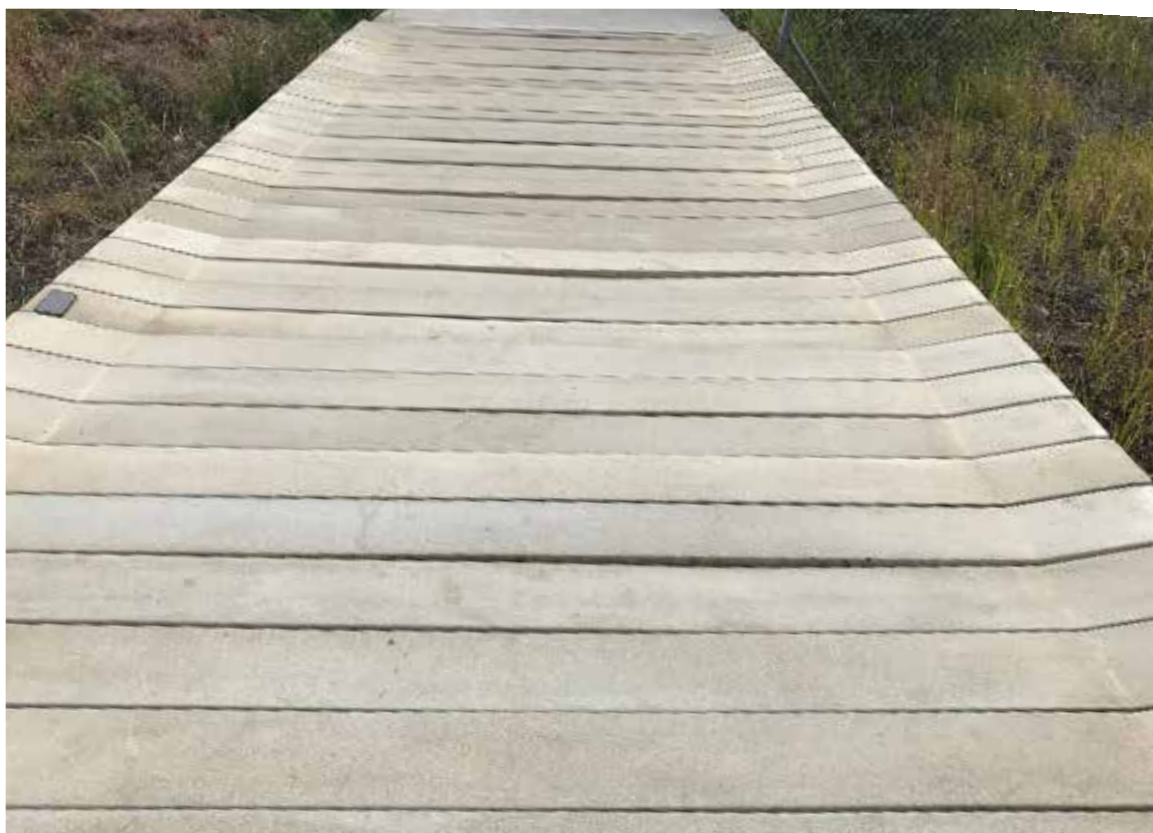
Low bridges over rain gardens
